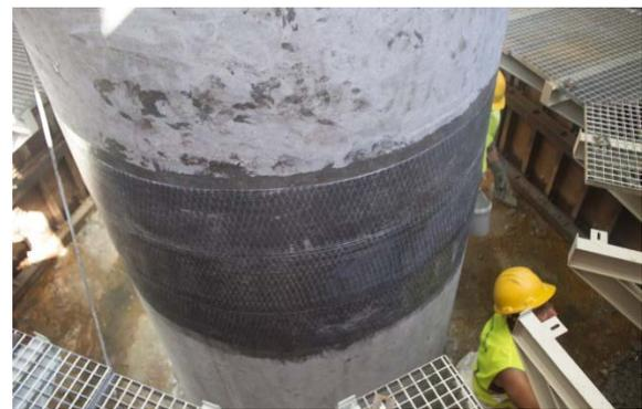
Repair (and protection) of Vasco da Gama Bridge columns with CFRP sheets [I.31]
