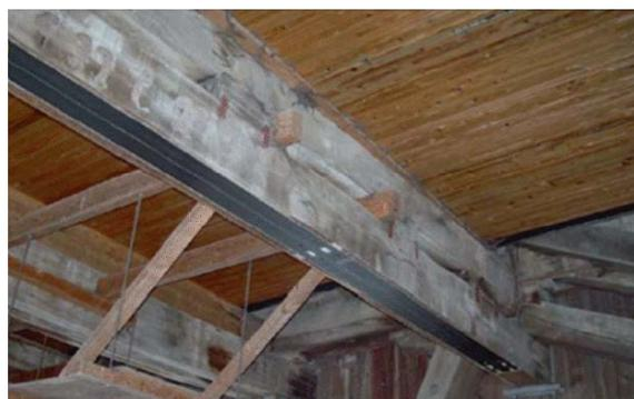
Strengthening of timber beams with CFRP laminates [I.32]
