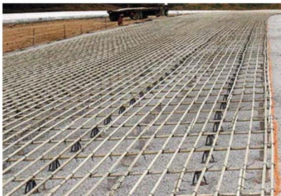
Reinforced concrete slab with GFRP rebars [I.30]
