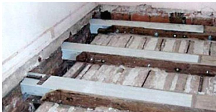
*Figure 2.13: GFRP pultruded profiles used in the rehabilitation of a timber floor [3].*
