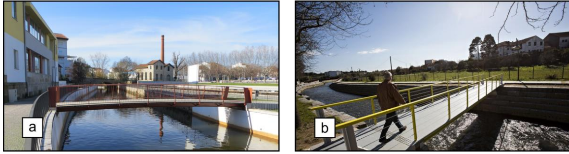
Figure 2.13. (a) S. Mateus, and (b) S. Silvestre pedestrian hybrid composite bridges [2.7, 2.34].
