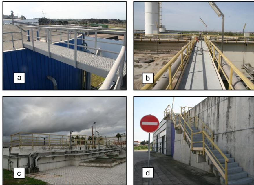
Figure 2.10. Handrails, and walkways made with pultruded GFRP components in Portuguese water treatment facilities (a) all-GFRP walkway, (b)-(c)-(d) handrails and staircases.
