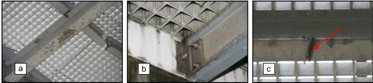
Figure 12.2. Anomalies: (a) surface marks; (b) biological colonisation and corrosion of metallic elements in the connections; (c) indentation in a transverse profile.
