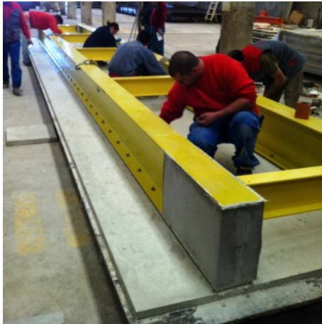
Figure 7.21.: Installation of the washers and nuts.
