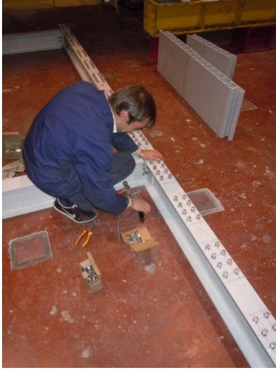
Figure 6.26.: Assembly of the main and secondary girders.
