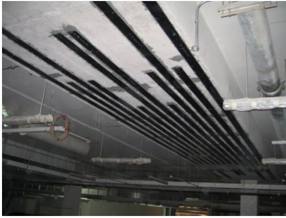
Figure 2.3.: CFRP flexural strengthening [22].
