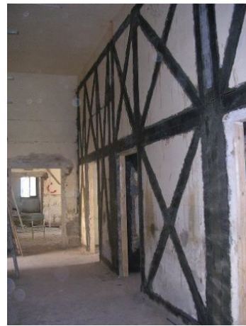
Figure 2.6.: CFRP strengthening of masonry structure [23].
