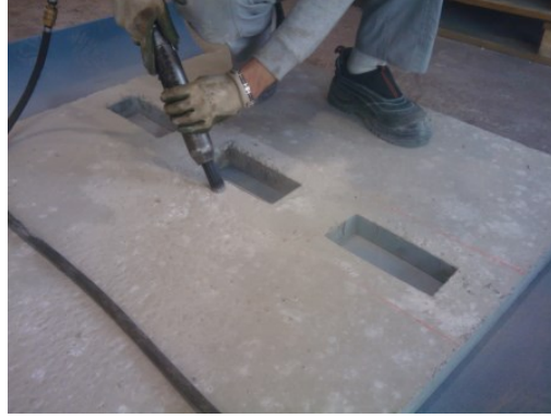
Figure 6.6.: Roughening of the slab (detail).
