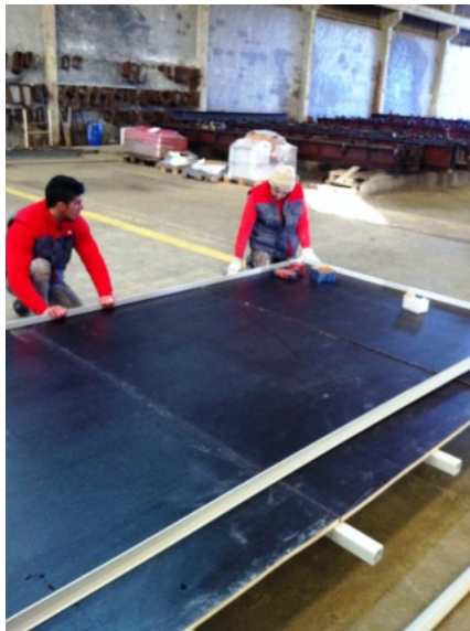
Figure 7.11.: Construction of the formwork.
