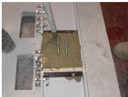
Figure 6.21.: Vibration of the concrete.
