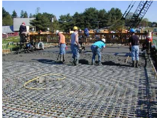
Figure 2.11.: Application of CFRP reinforcement bars [28].
