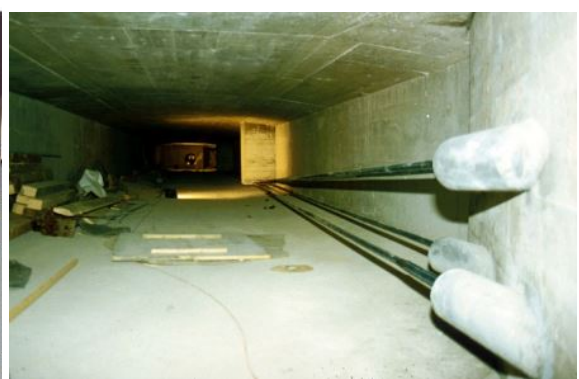
Figure 2.8.: CFRP prestress cables [24].
