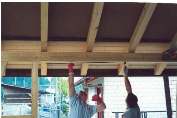
Figure 2.7.: CFRP strengthening of timber structure [22].
