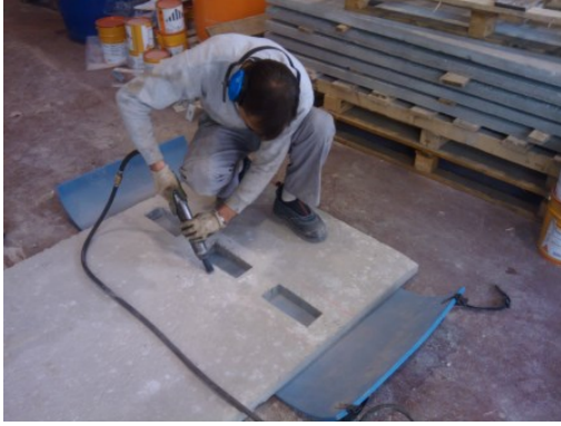
Figure 6.5.: Roughening of the slab.
