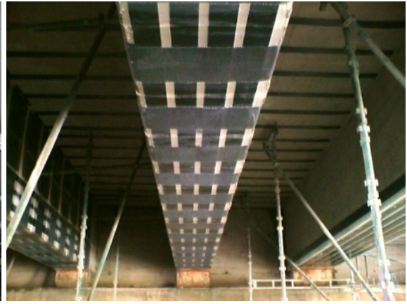
Figure 2.4.: CFRP shear strengthening [22].
