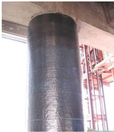
Figure 2.5.: CFRP axial strengthening [22].
