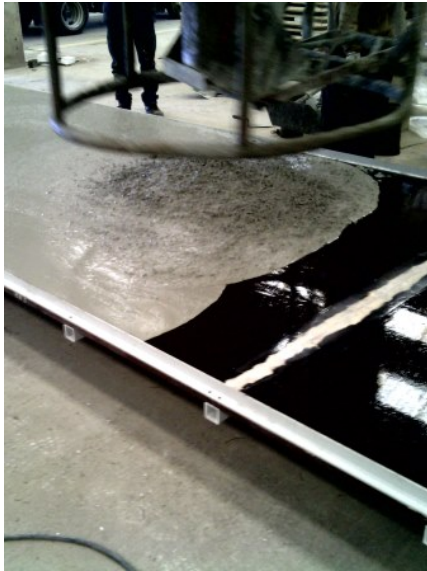
Figure 7.13.: Casting of the SFRSCC slab.
