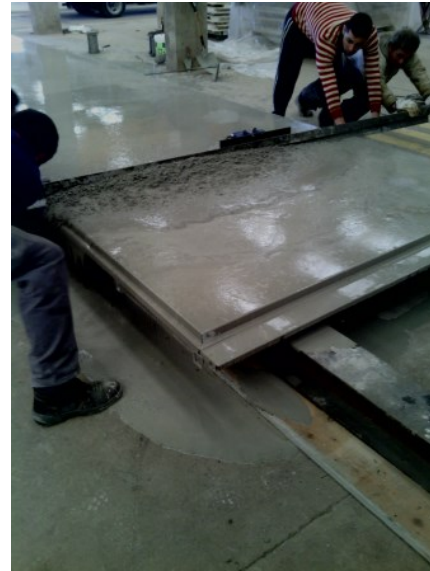
Figure 7.14.: Regularization of the slab surface.
