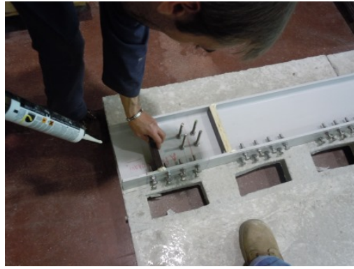
Figure 6.17.: Installation of the formwork.
