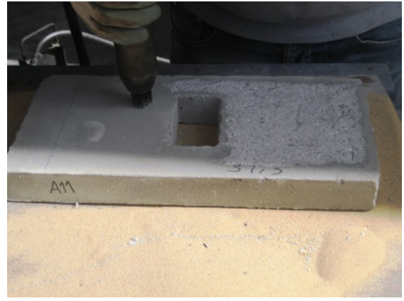
Figure 5.10.: Surface preparation of a SFRSCC slab (with negative) for the adhesive bonding.
