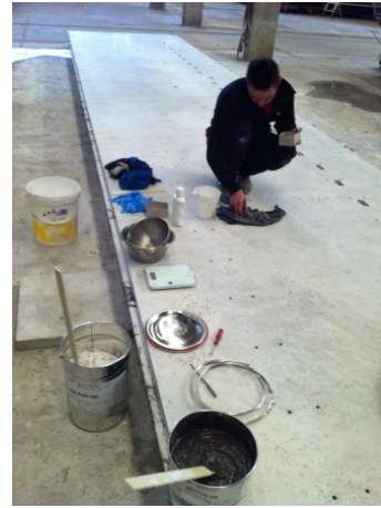
Figure 7.18.: Installation of the stainless steel connectors.
