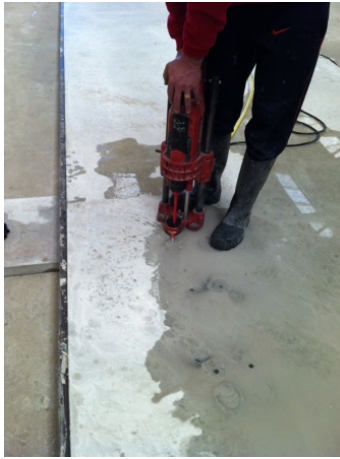
Figure 7.17.: Drilling of the SFRSCC slab.
