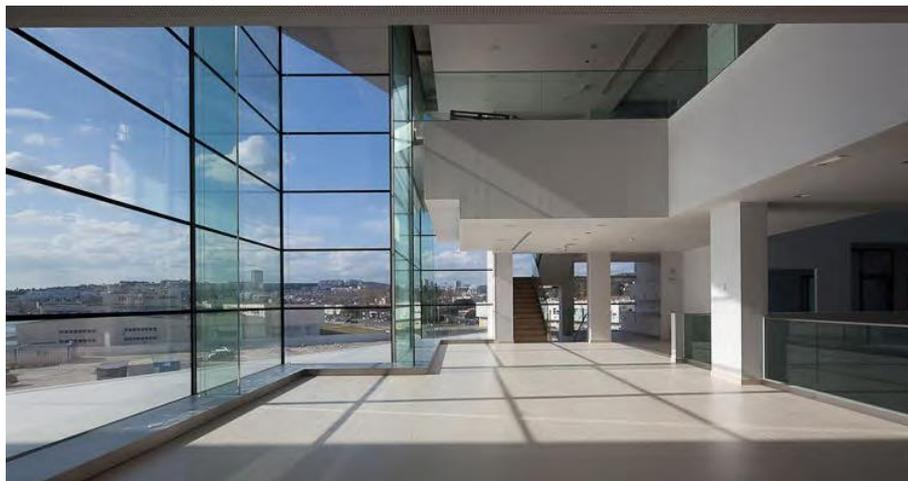
Fig. 3.1 – *Champalimaud Centre for the Unknown* building facade and its glass fins (courtesy of José Campos).
