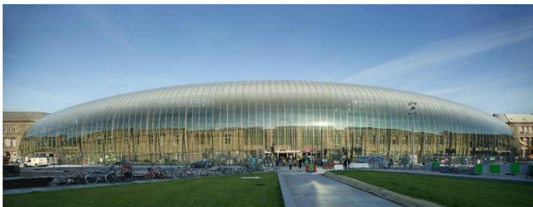
Fig. 2.34 – Cold bent laminated glass panels applied in the Strasbourg train station [2.103].
