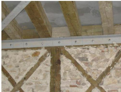
Figure 7.1. Connection between a timber floor and timber-framed masonry walls using steel angles.
