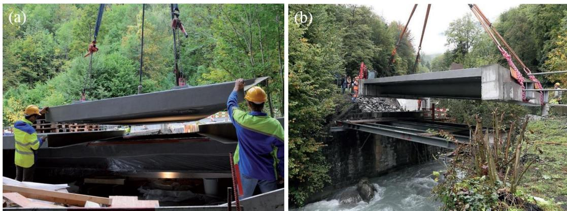
Figure 2.5. Avançon River bridge deck near Bex, Switzerland [7]: (a) assembly of the deck components on the river bank, and (b) placement of the deck.
