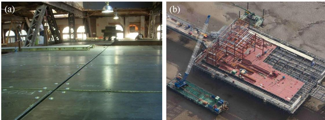
Figure 2.2. Heavy duty sandwich panels with steel facings and solid elastomer cores: (a) in-fill floor at the Carnegie Hall (Manhattan, New York, USA) [3], and (b) Grand Pier in Weston-super-Mare (UK) [4].
